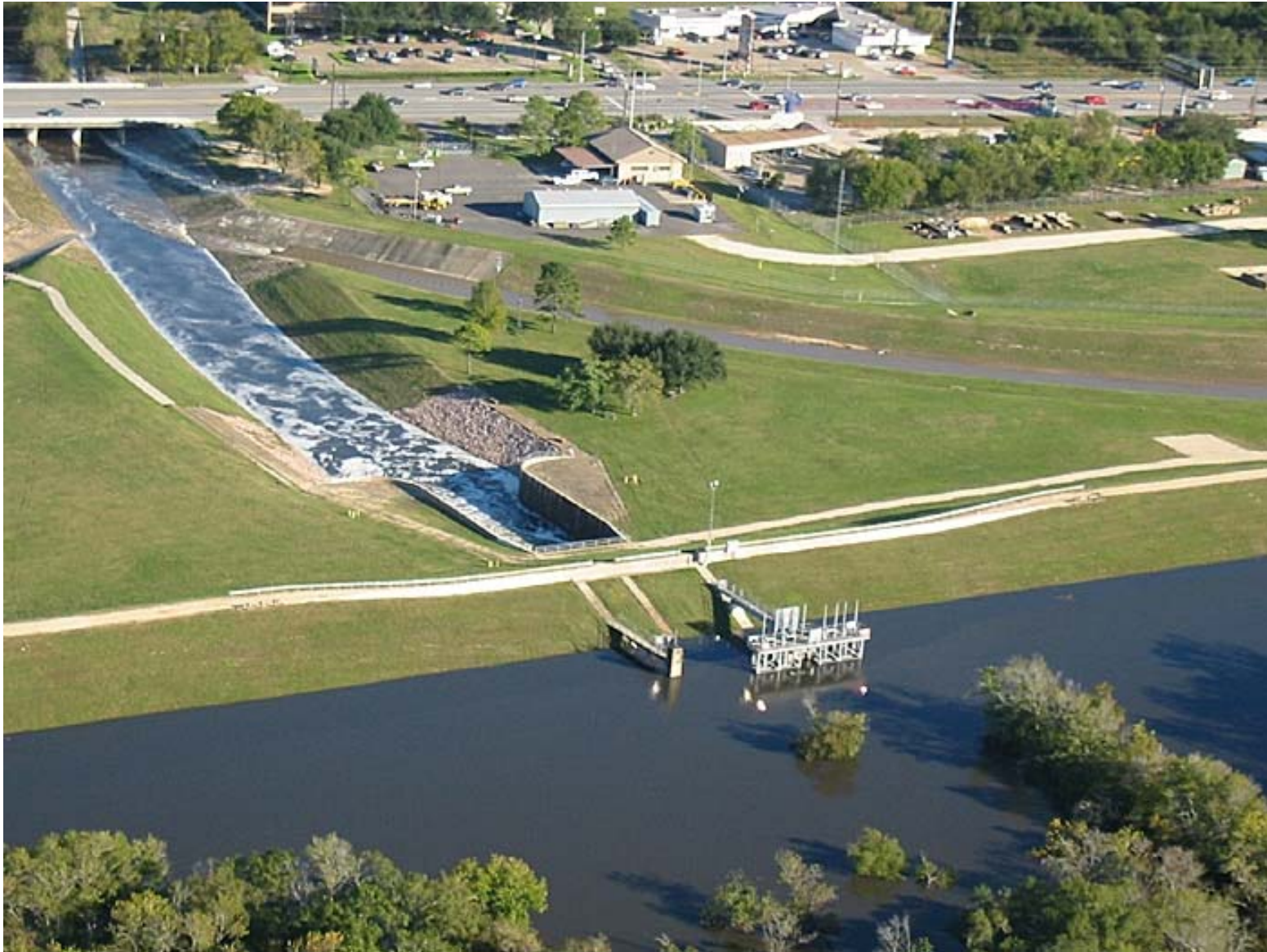
BARKER RESERVOIR – OUTLET WORKS
