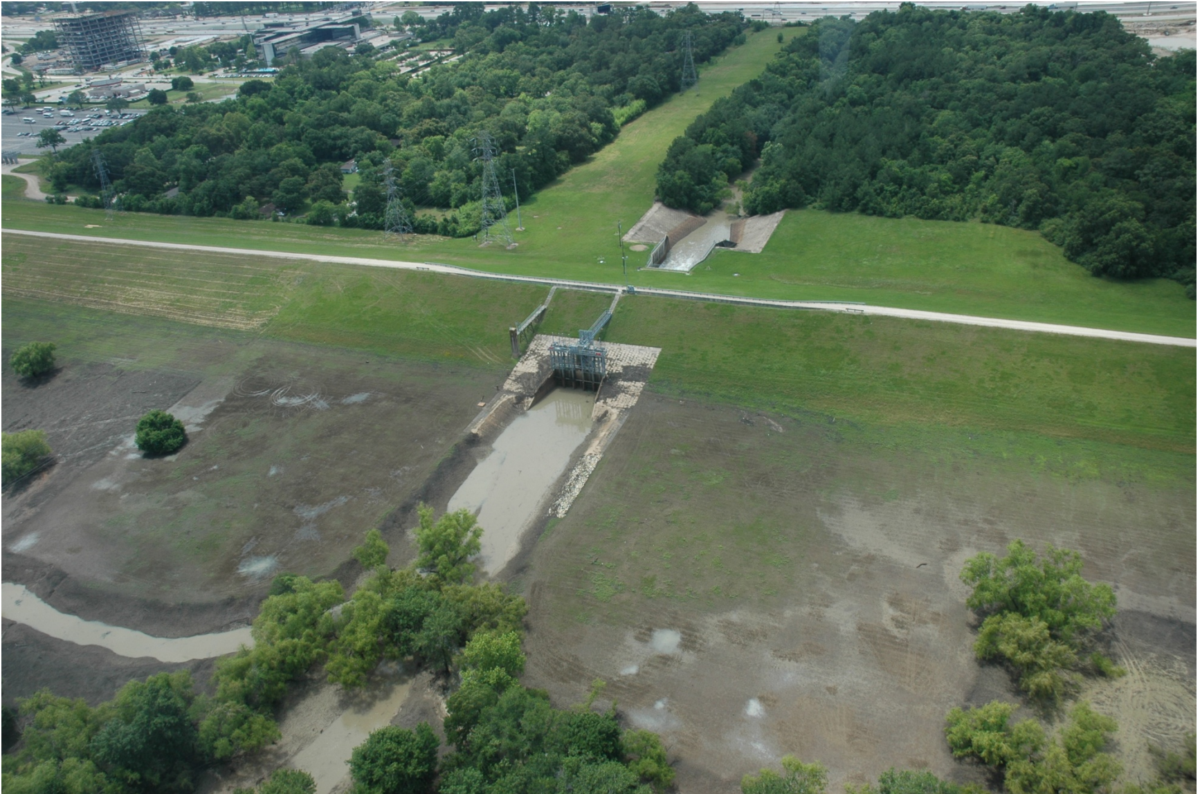
ADDICKS RESERVOIR – OUTLET WORKS
